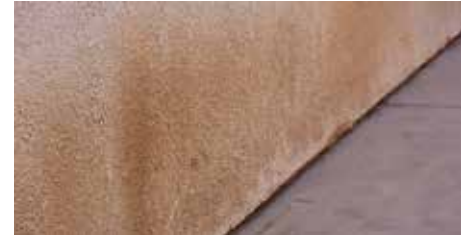
Permanent stains on stucco wall - wall needs painting
