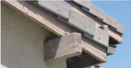
Weathered and split fascia will soon need to be replaced
