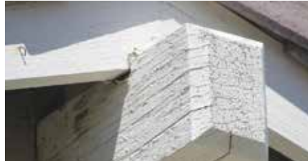
Weathered and worn end beam is beginning to split
