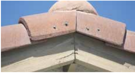
Fascia boards beginning to split due to lack of caulking
