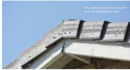
No caulking where fascia boards meet allowed them to warp
